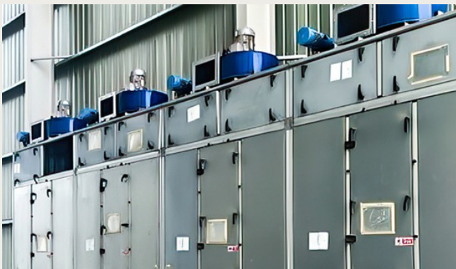
AGI PTM intake and filtration system.
