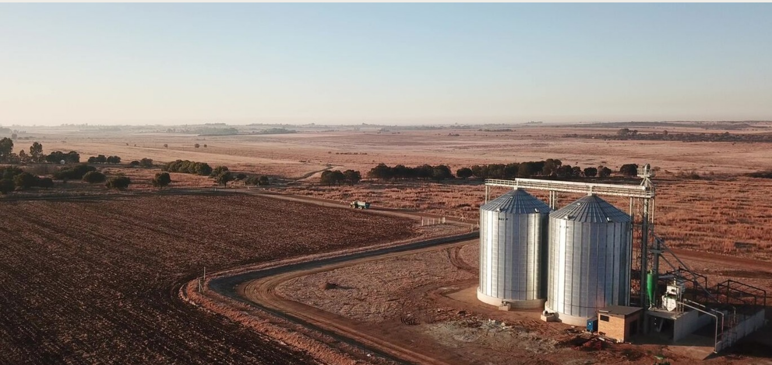
Grain facility. Photograph: AGI.
