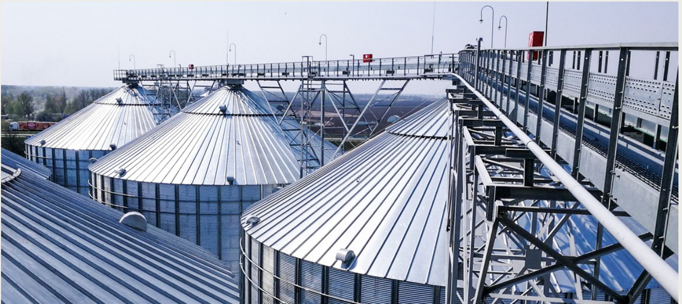
Catwalks and support structures. Photograph: AGI.
